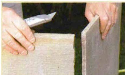
3. The board should break cleanly. Once fibers on the back of the board have been severed, the sheet should break cleanly along the score line.
